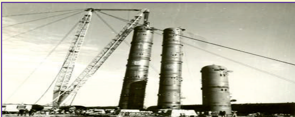
Kota Plant 4.5 m dia x 53 m ht x 286 T Exchange Tower erection
